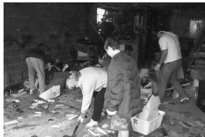
First Bethel team shovels debris from SHIM garage.
